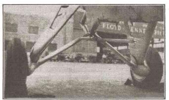
The Vought SBU-2's bomb release "crutch" is shown in this interesting undercarriage close-up. Note the clean streamlining about the metal fittings of the landing gear legs. All military plane parts must be both staunch and trim.
